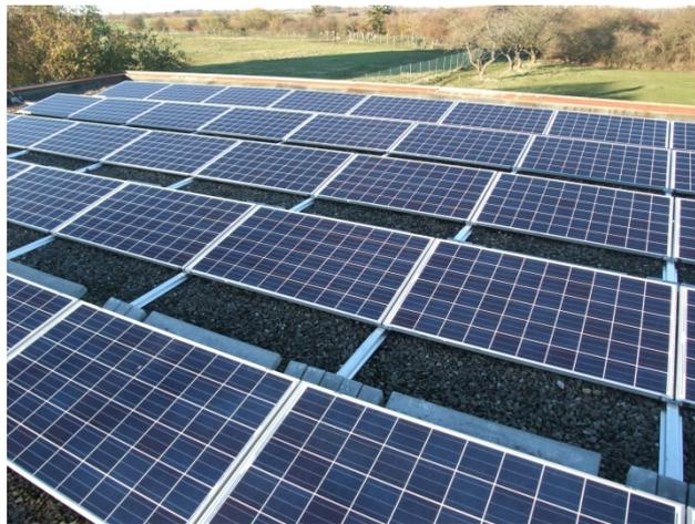
Statkraft's first solar park in Germany was constructed in 2018, next to the hydropower plant in Dörverden. The 750 kW park is a test site for the combination of solar power and batteries.
