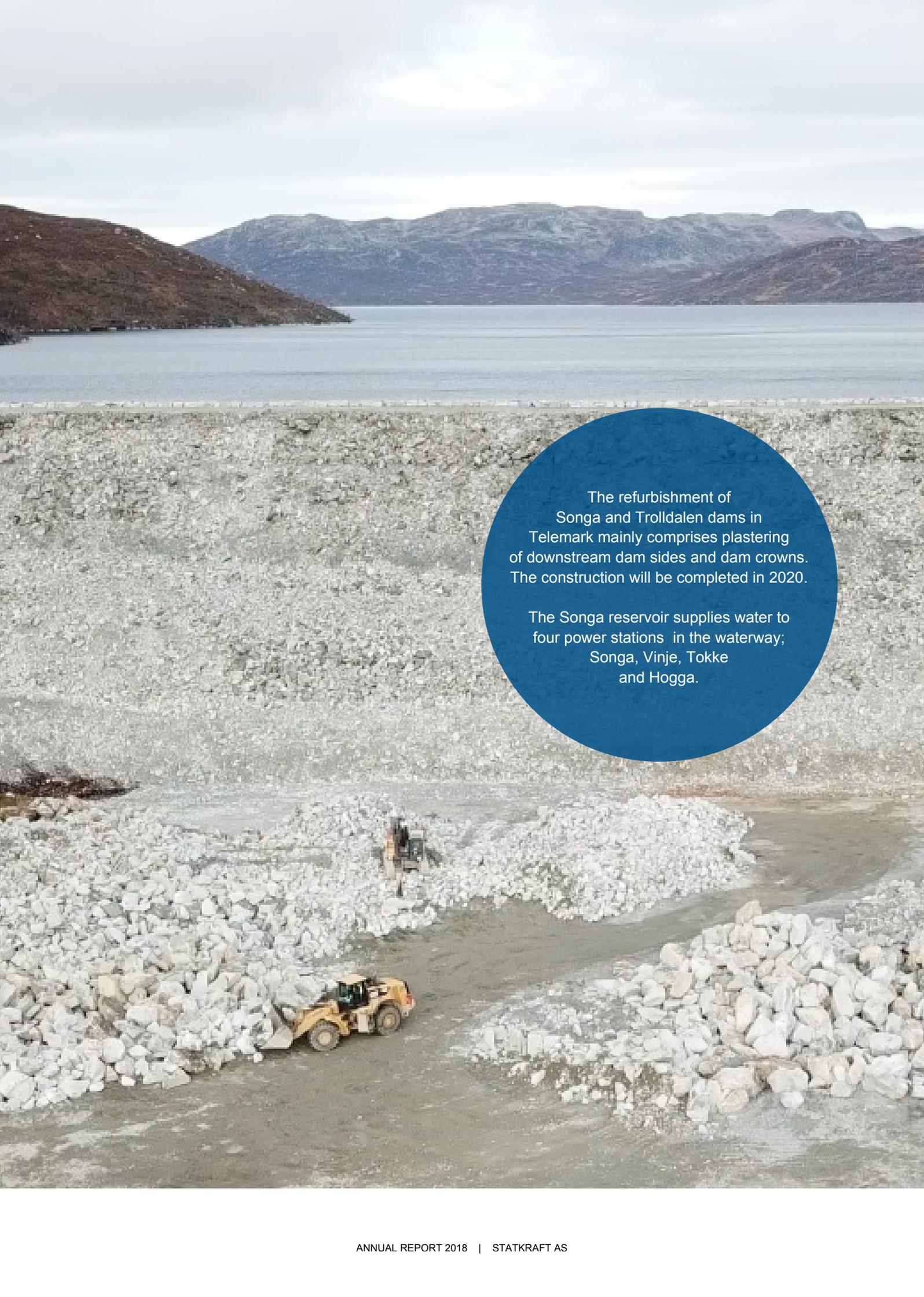
The refurbishment of Songa and Trolldalen dams in Telemark mainly comprises plastering of downstream dam sides and dam crowns. The construction will be completed in 2020.
